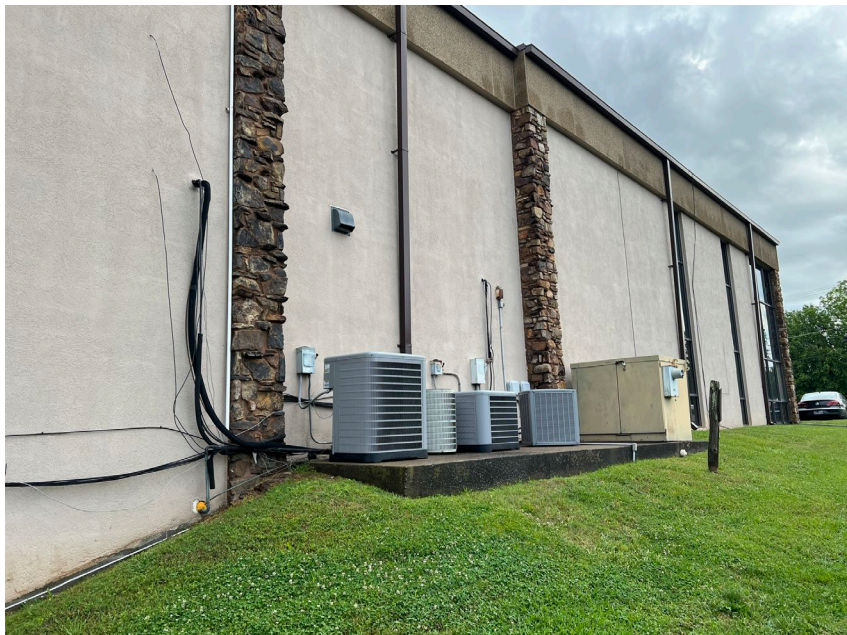
Photo #2 – South Elevation of Structure
