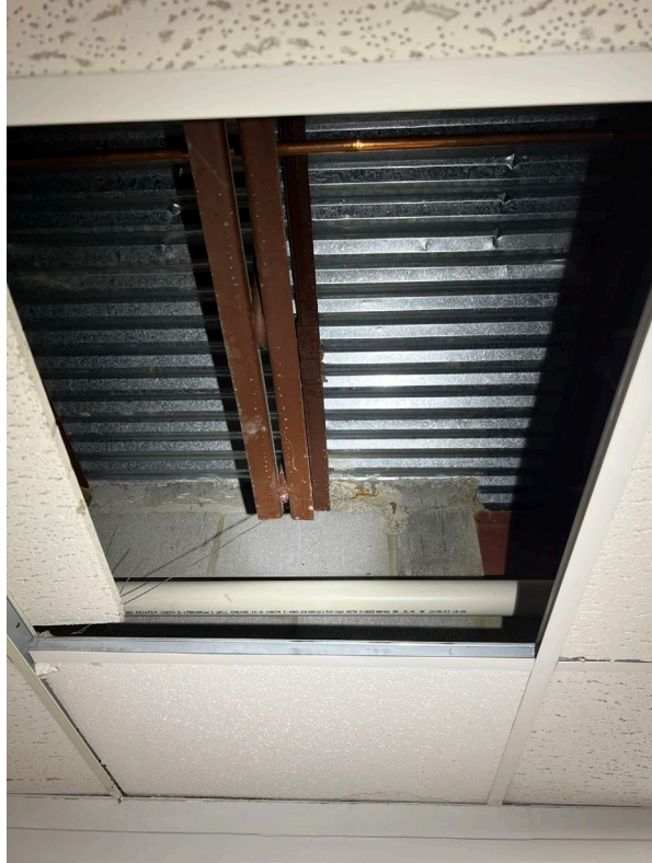
Photo #5 – Above Ceiling Framing
