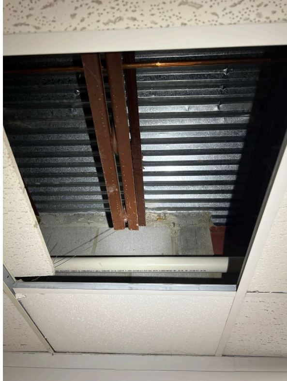
Photo #5 – Above Ceiling Framing
