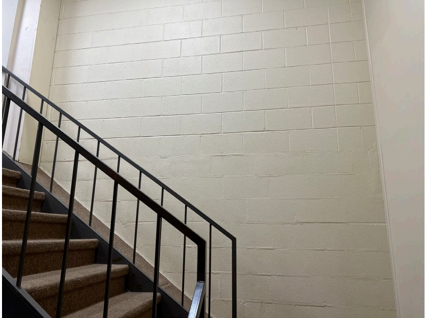
Photo #3 – CMU in Stairwell
