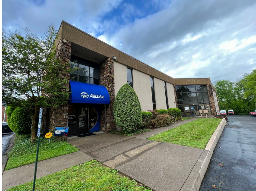
Photo #1 – North Elevation of Structure
