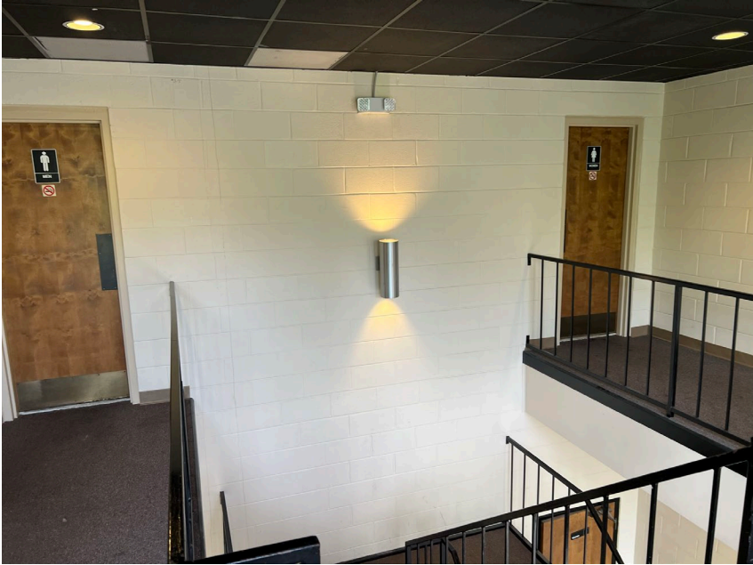
Photo #4 – Monumental Stairwell
